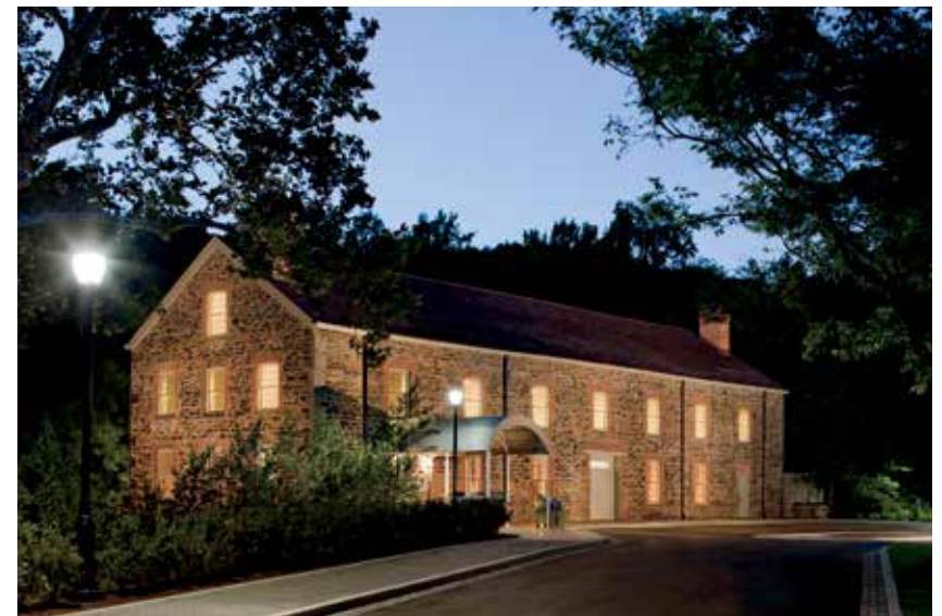
The restored Goldman Stone Mill. Photo © Robert Benson Photography.
