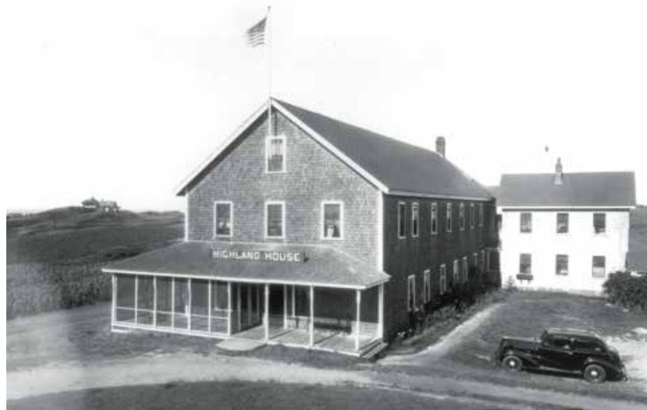
Fig. 10.4. Highland House, Truro, c. 1935. NPS.
