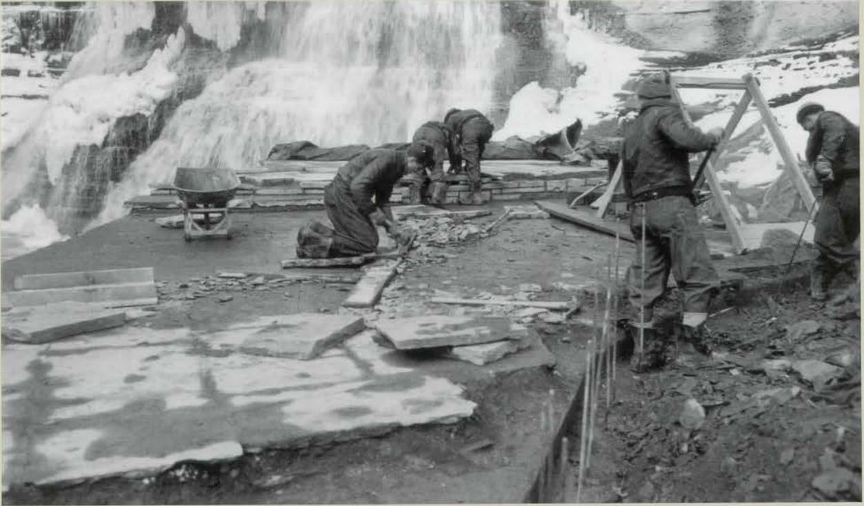
Civilian Conservation Corps masons at work creating viewing platform at Lucifer Falls. Courtesy New York State Office of Parks, Recreation and Historic Preservation, Finger Lakes Region.
