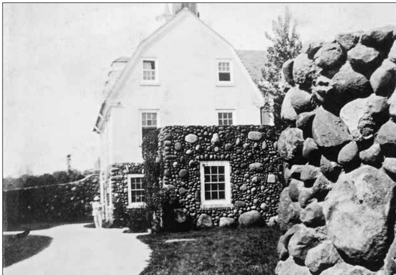
Foundation of the dairy and retaining wall.
