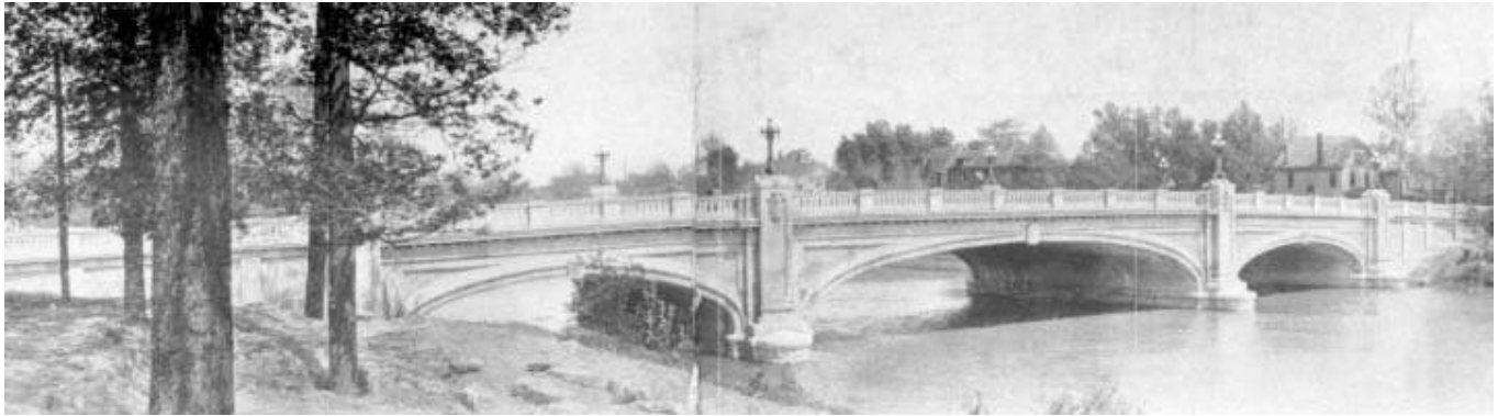
Bridge on Capitol Avenue, Indianapolis. Park and boulevard system by George Kessler. Courtesy Storrow Kinsella Associates.
