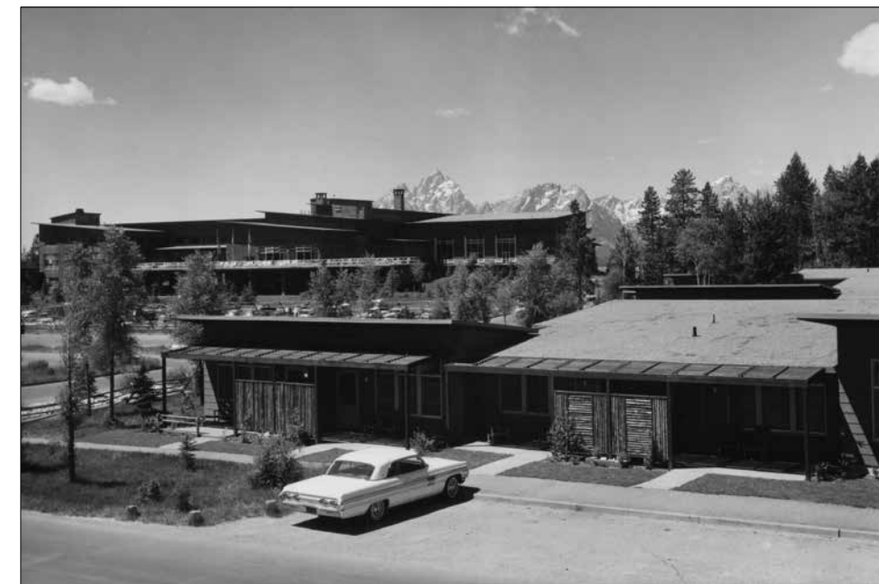
The Jackson Lake Lodge featured decentralized motel units as well as the main lodge building. NPS Historic Photo Collection.
