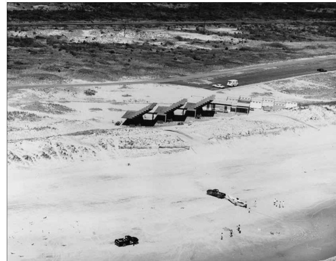
Coquina Beach bathhouse and shade structure, Cape Hatteras National Seashore, designed by the EODC in 1955. NPS Historic Photo Collection.
