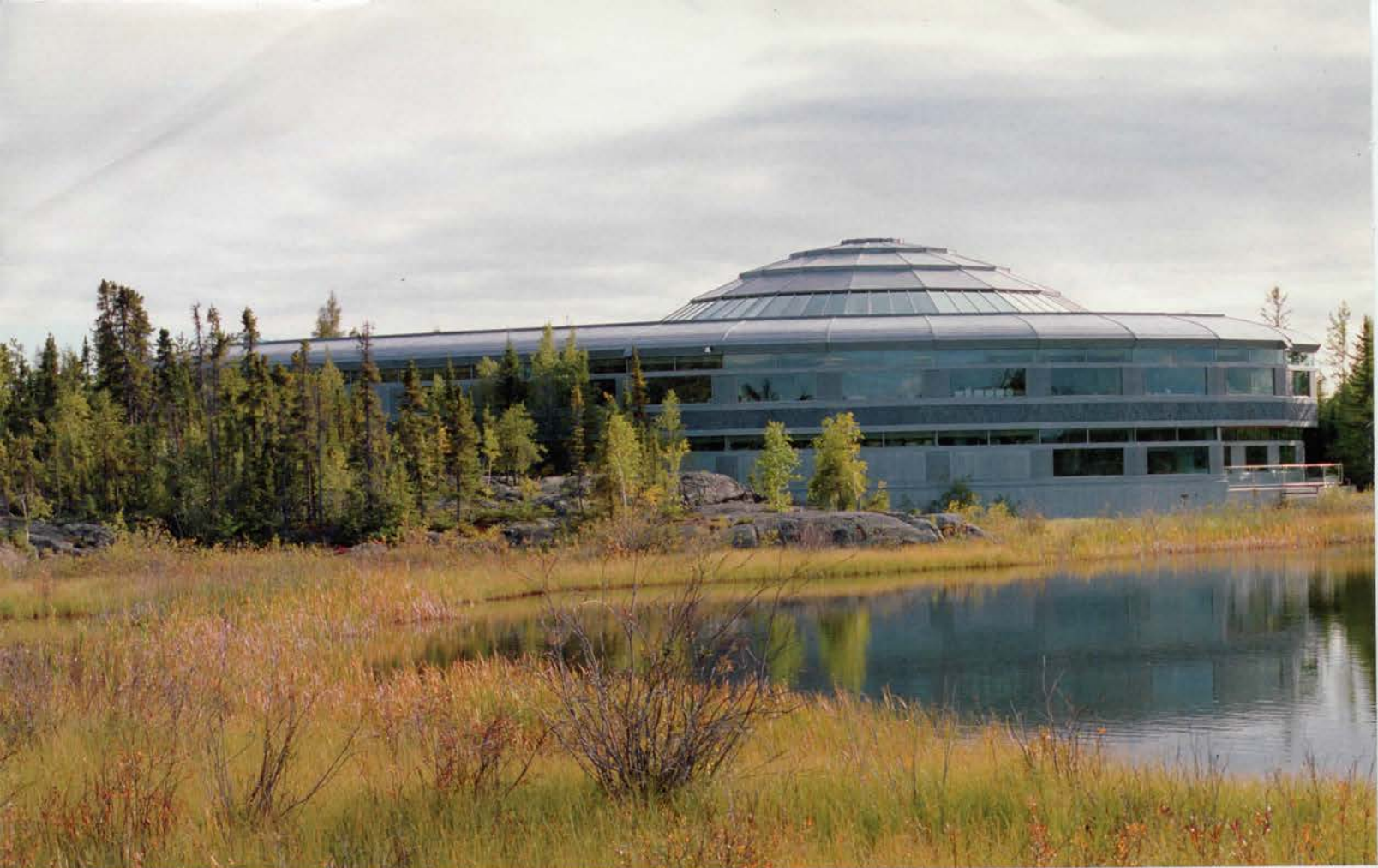
Northwest Territories Legislative Assembly Building in Yellowknife, Canada. Photograph by Etta Gerdes ©.
