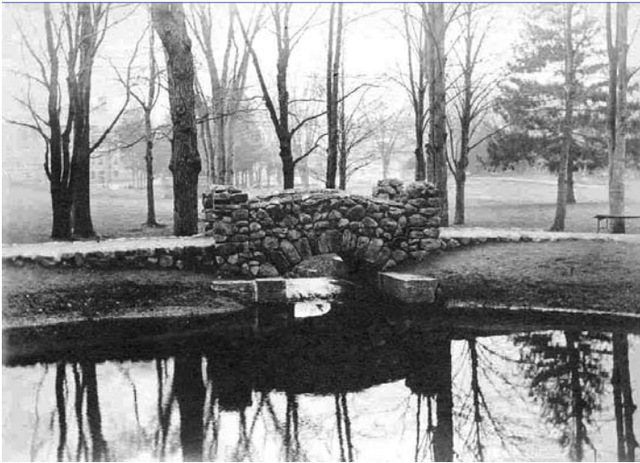
Stone bridge in Wilcox Park, designed by Manning, 1905. Historic photo courtesy of Elmore Design Collaborative.
