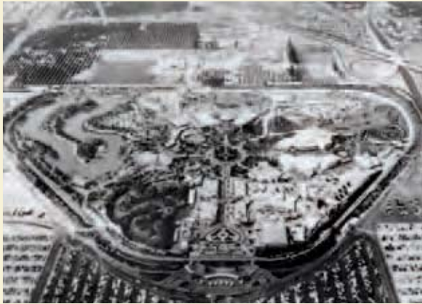
Aerial view of Disneyland, 1956. USC Regional Historical Photo Collection. Wikimedia Commons.
