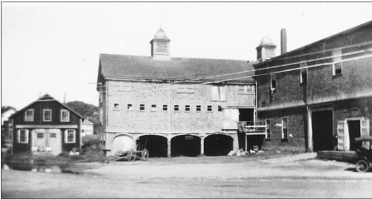
Figure 18. The train station was a primary gateway to Cohasset, Massachusetts, and the Tilden stables pictured here were just across the street. Once they were acquired and demolished Nolen designed a small park for the site. Cohasset Historical Society .
