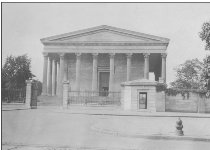
Figure 2. The main building at Girard College, the school for orphans where Nolen lived and studied from 1878 until 1887. Nolen Papers, Cornell University Library.
