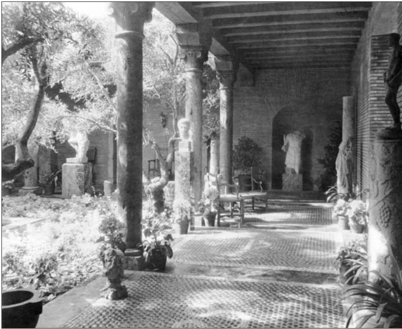
13.15. Courtyard with classical sculpture, guesthouse. Courtesy Kellam de Forest.
