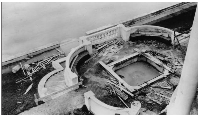
3.4. Construction of fountain terrace, 1907. Gwinn.
